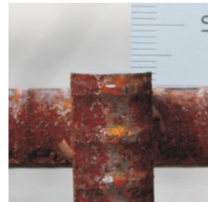
Rebar rod can be cut flush to a surface, with only 2-3mm showing
